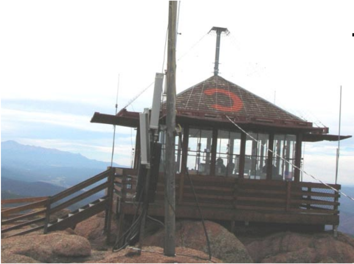
Figure 14 - Devil's Head Fire Lookout Tower (AP Sector Antennas in Foreground)
